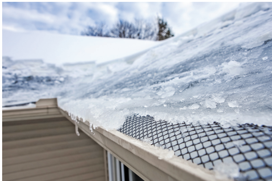
WINTER PROBLEM – Ice dams form in a gutter, potentially causing serious damage to the home. Image: soupstock. Adobe Stock.
